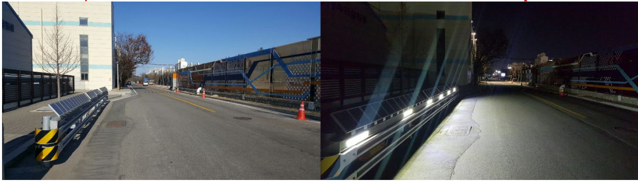
Figure 1: Low lighting system(left:daytime, right:nighttime)
